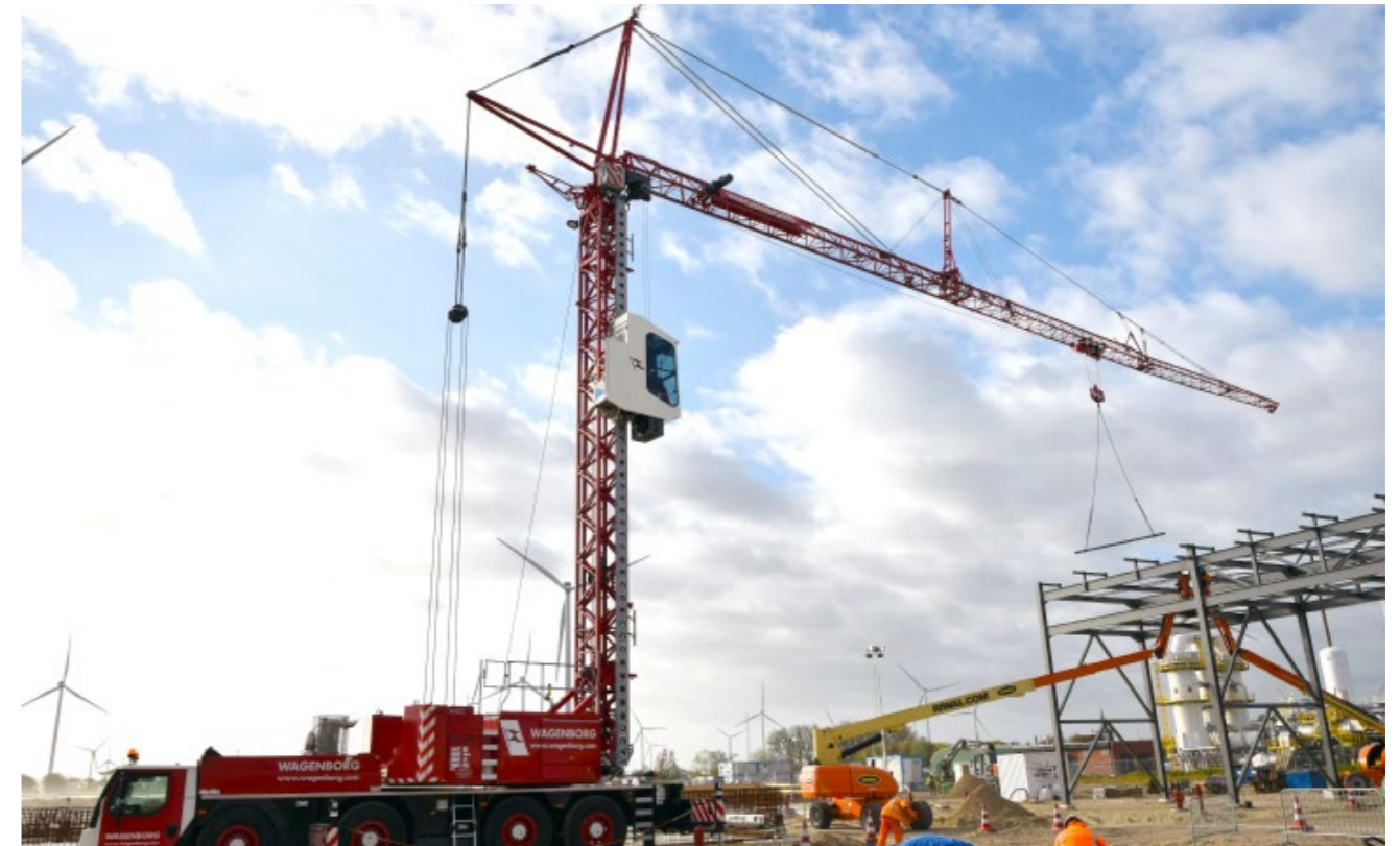
Mobile towercrane Liebherr
