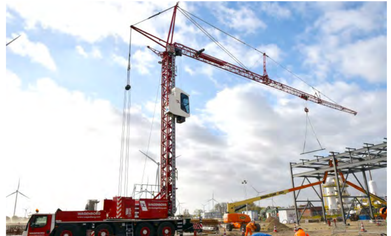
Mobile towercrane Liebherr
